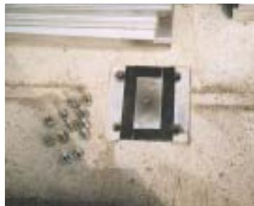
**BLOBEL Flood Protection Systems are designed to withstand high water pressure. The double U-shaped steel columns are mounted on anchor plates, which are set in a concrete footing.**
