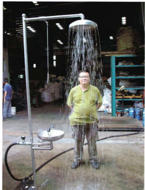
Shower head give a concertrated flow of water in a drench colum with radius of 200mm comply to ANSI 2358.1-2004.
